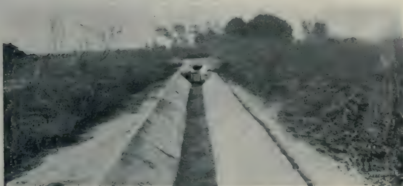
Subsidiary Channel—about 18 inches at bottom. (Lined with concrete.)
